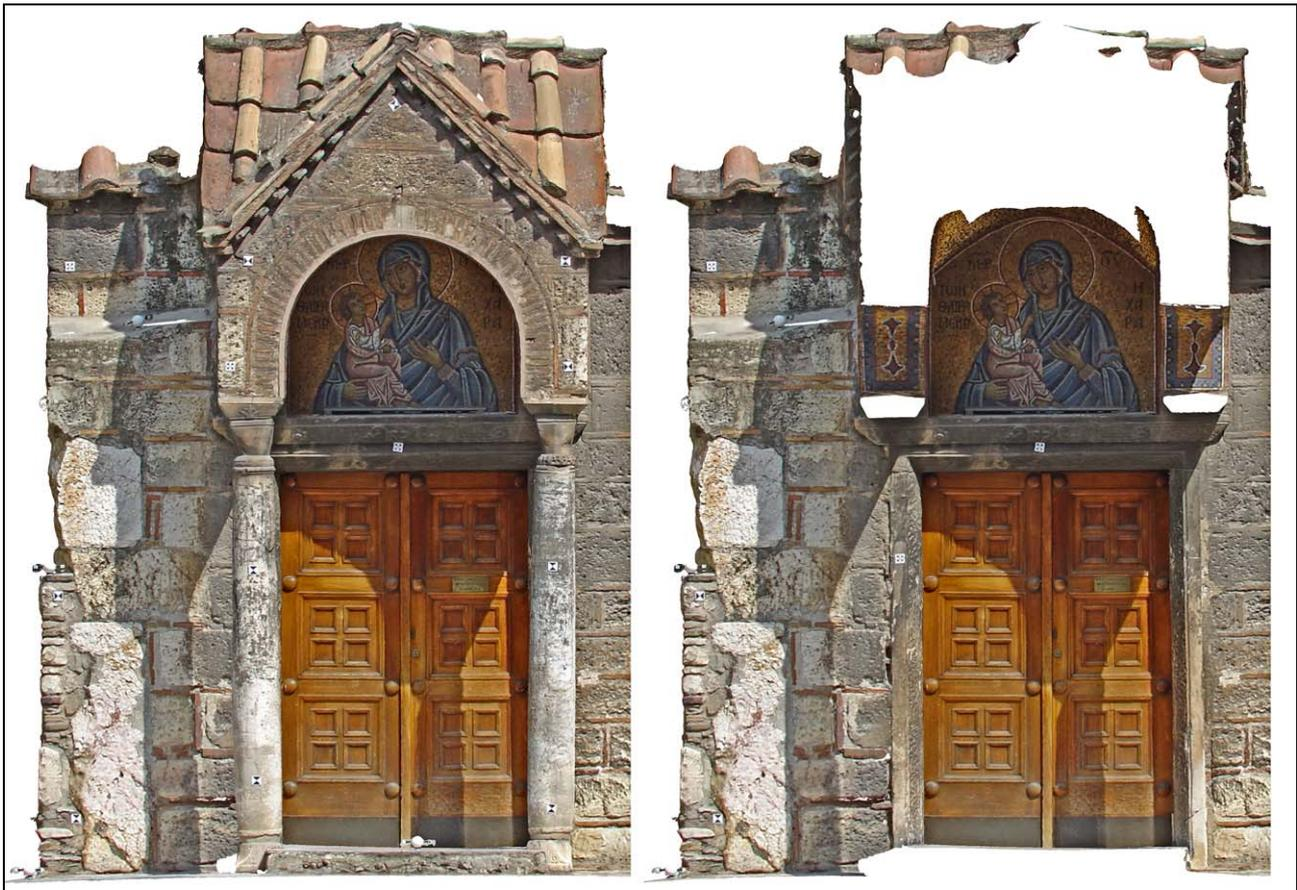
Figure 8. Left: Extract of the orthoimage from 7 images. Right: orthoprojection of a model section defined by a maximum Z-value.
