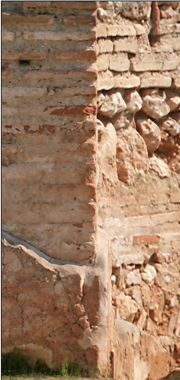
Figure 15. Detail of orthoimage, generated by blending texture from 9 images, in the area of an object edge.
