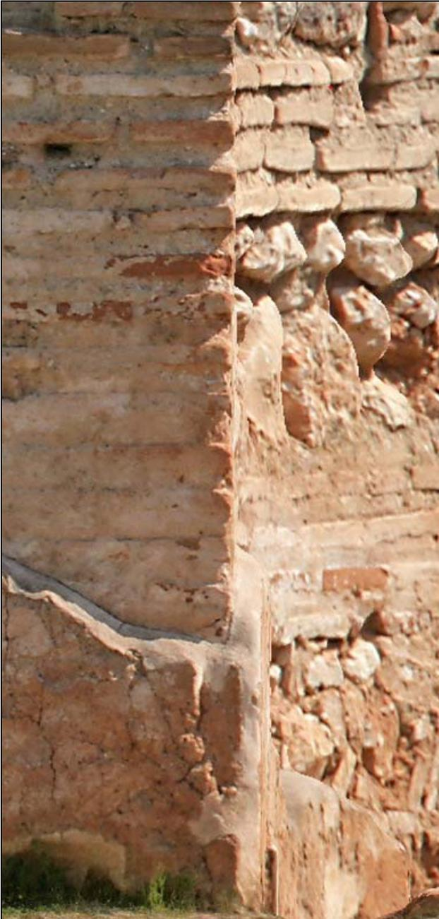
Figure 10. Orthoimage detail of part 1 generated by blending texture from 9 images.
